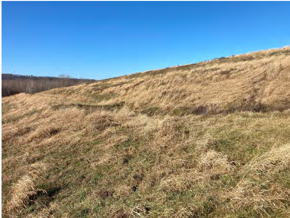
Photograph 12: Non-contact stormwater channel on south slope is clear of obstructions. The final cover south slope is well vegetated and mowed annually. No evidence of animal burrows, erosion, or stability issues.
