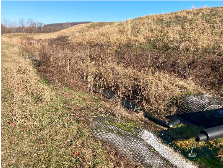
Photograph 17: West non-contact stormwater channel looking north is clear of obstructions. West final cover lower slope is well vegetated and mowed annually. No evidence of animal burrows, erosion, or stability issues.
