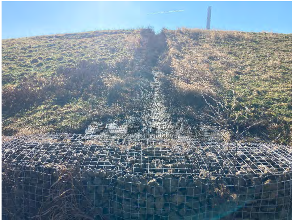
Photograph 23: Non-contact stormwater downchute in northeast corner is clear of obstructions. Gabion energy dissipator is installed at the junction with the stormwater (non-contact water) perimeter ditch.
