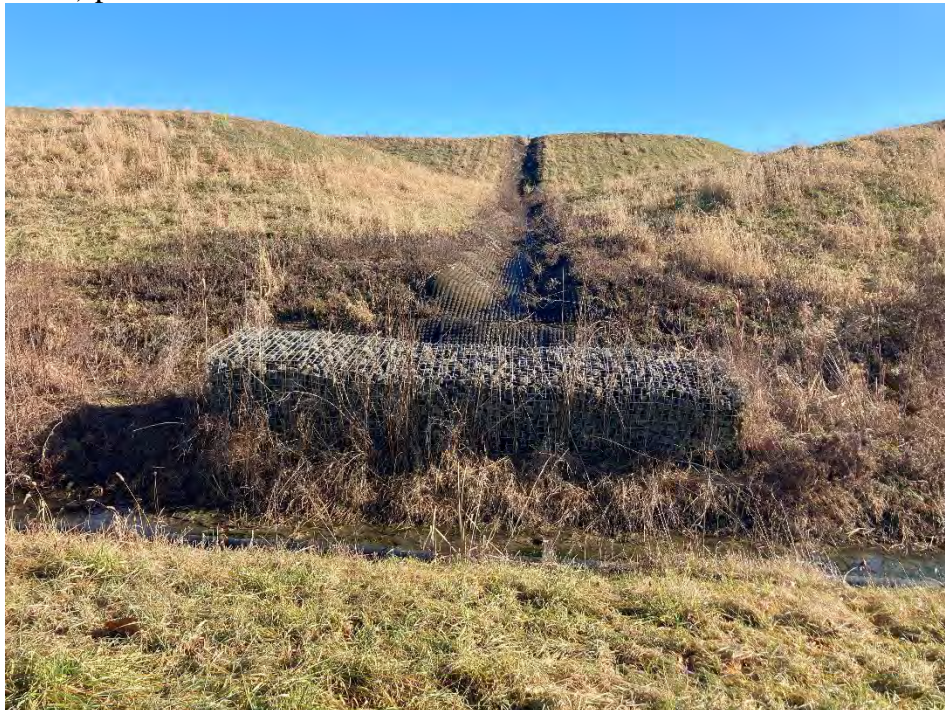
Photograph 28: Non-contact stormwater downchute on west slope is clear of obstructions. Gabion energy dissipator is installed at base of downchute before the stormwater perimeter ditch.
