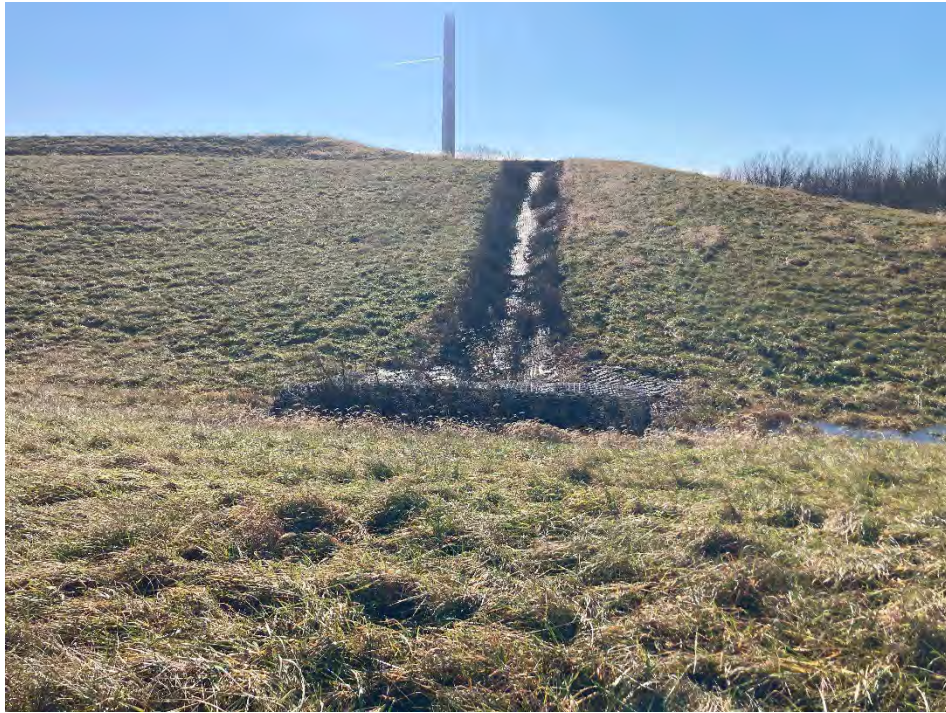
Photograph 21: Non-contact stormwater downchute in northwest corner is clear of obstructions. Gabion energy dissipator is installed at the junction with the stormwater (non-contact water) perimeter ditch.
