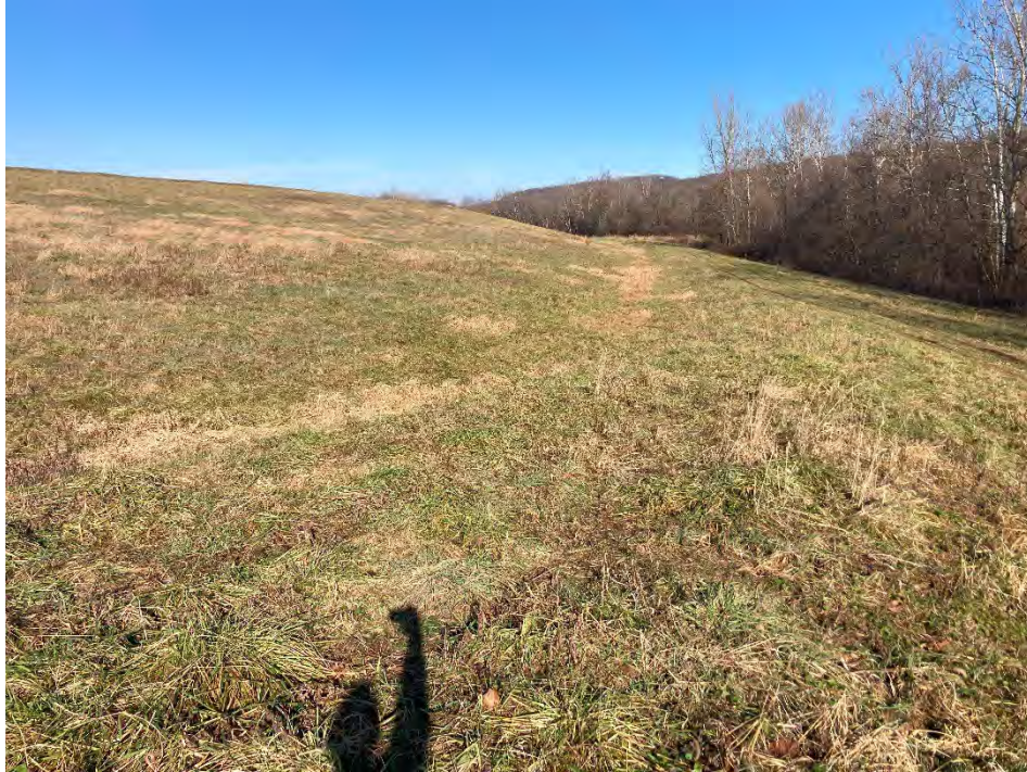
Photograph 25: East non-contact stormwater channel looking north is clear of obstructions. East final cover lower slope is well vegetated and mowed annually. No evidence of animal burrows, erosion, or stability issues.
