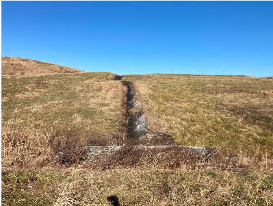
Photograph 27: Non-contact stormwater downchute on south slope is clear of obstructions. Gabion energy dissipator is installed at the junction with the stormwater (non-contact water) perimeter ditch.
