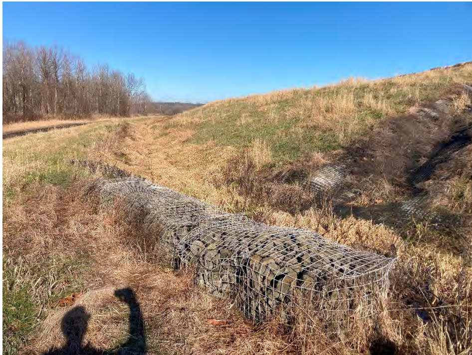
Photograph 14: West non-contact stormwater channel looking north is clear of obstructions. West final cover lower slope is well vegetated and mowed annually. No evidence of animal burrows, erosion, or stability issues.
