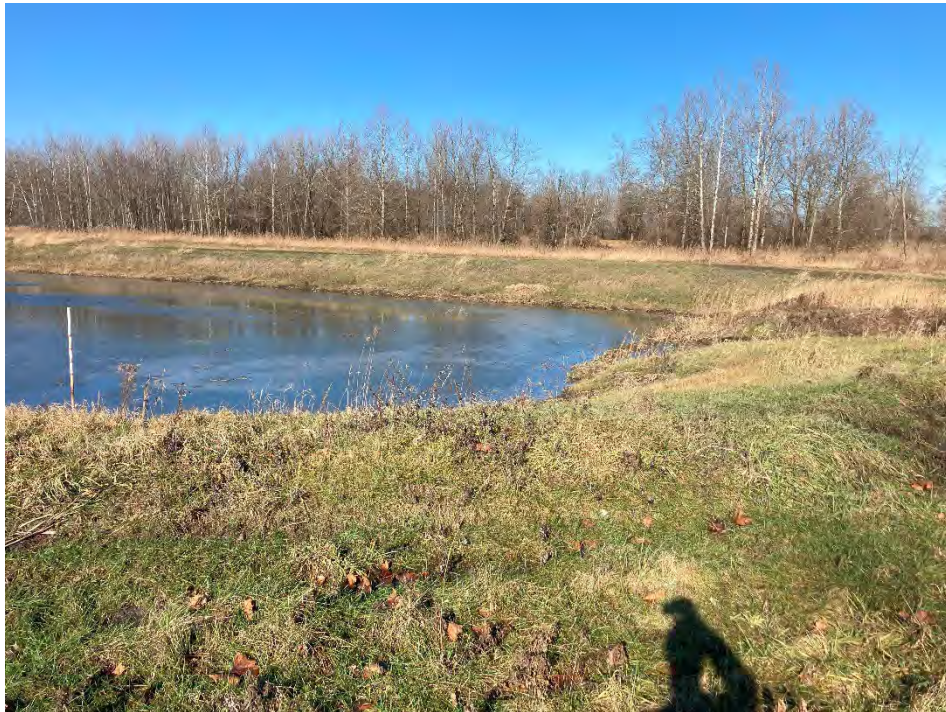
Photograph 18: Leachate (contact water) Pond. No evidence of animal burrows or liner damage.
