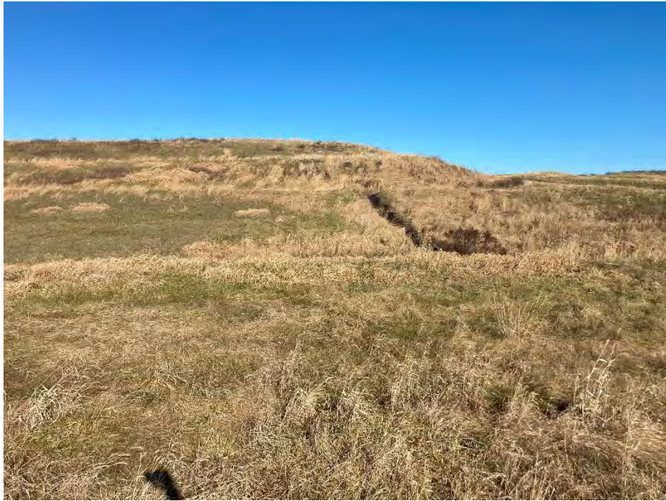
Photograph 11: Non-contact stormwater downchute on south slope is clear of obstructions. Gabion energy dissipator is installed at the junction with the stormwater (non-contact water) perimeter ditch.
