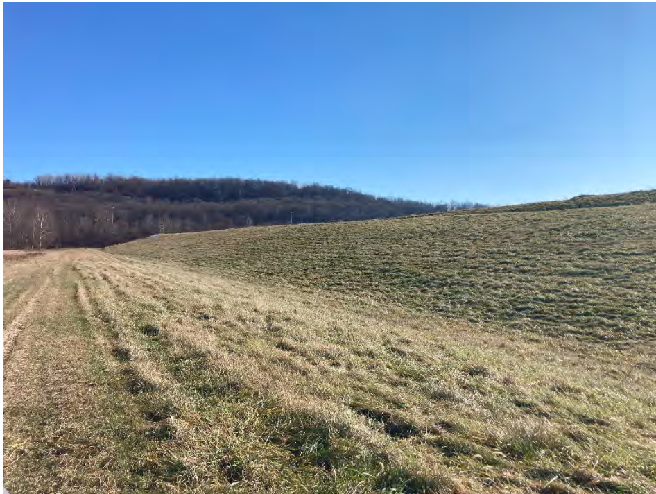
Photograph 22: North non-contact stormwater channel is clear of obstructions. North final cover lower slope is well vegetated and mowed annually. No evidence of animal burrows, erosion, or stability issues.
