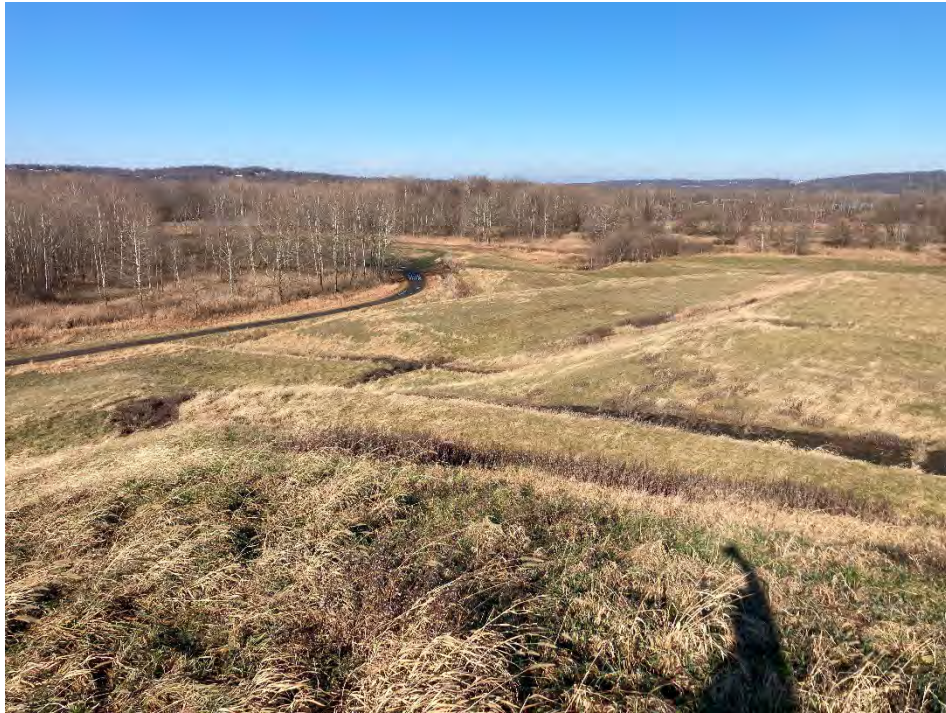
Photograph 4: Downchutes from west side of Stage 4 and Stage 5. No evidence of animal burrows, erosion, or stability issues.
