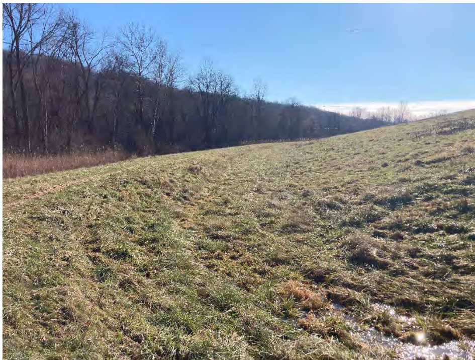
Photograph 24: East non-contact stormwater channel looking south is clear of obstructions. East final cover lower slope is well vegetated and mowed annually. No evidence of animal burrows, erosion, or stability issues.
