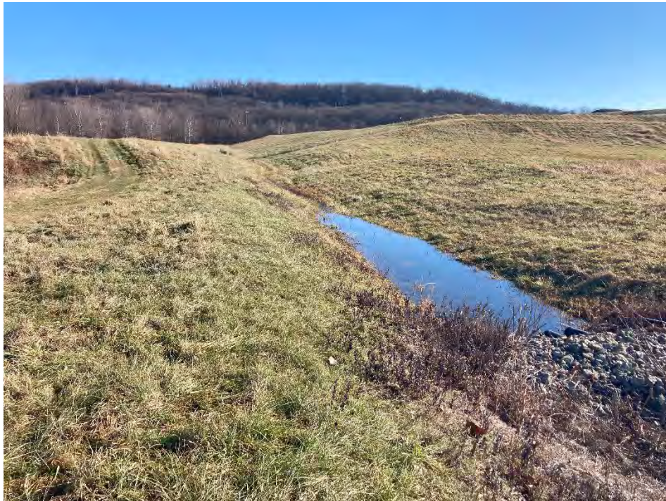
Photograph 20: North non-contact stormwater channel is clear of obstructions. North final cover lower slope is well vegetated and mowed annually. No evidence of animal burrows, erosion, or stability issues.
