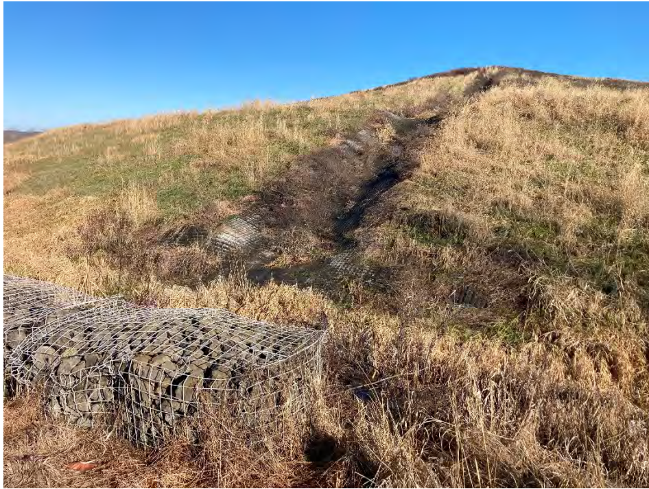
Photograph 13: Non-contact stormwater downchute in southwest corner is clear of obstructions. Gabion energy dissipator is installed at junction with the stormwater perimeter ditch.
