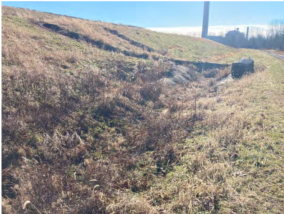
Photograph 15: West non-contact stormwater channel looking south is clear of obstructions. West final cover lower slope is well vegetated and mowed annually. No evidence of animal burrows, erosion, or stability issues.
