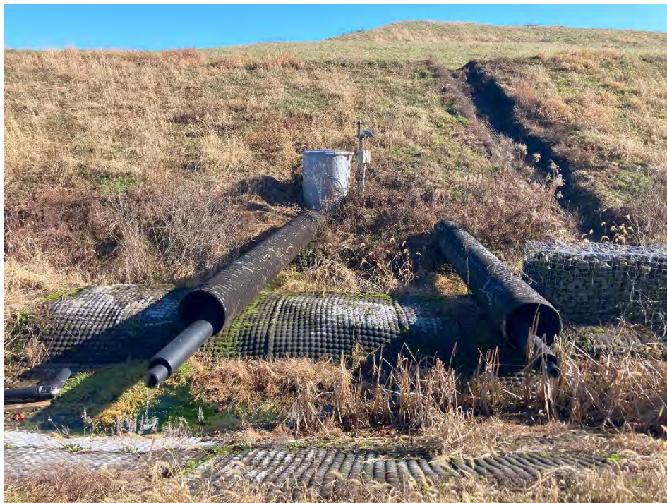
Photograph 16: Leachate collection zone and leak detection zone discharge pipes.
