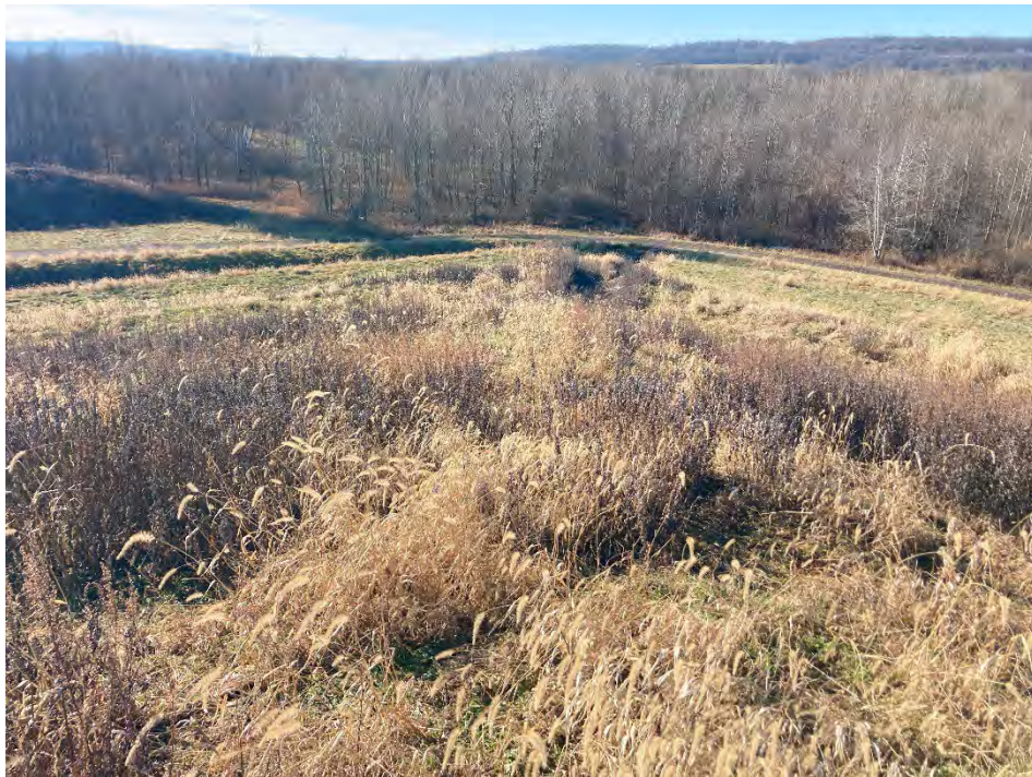
Photograph 6: Stage 4 southwest corner slope and downchute is well vegetated and mowed annually. No evidence of animal burrows, erosion, or stability issues.
