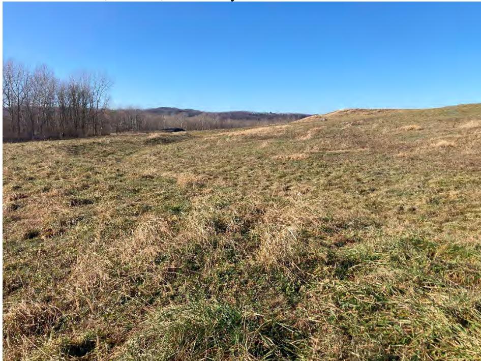
Photograph 26: South non-contact stormwater channel looking west is clear of obstructions. South final cover lower slope is well vegetated and mowed annually. No evidence of animal burrows, erosion, or stability issues.
